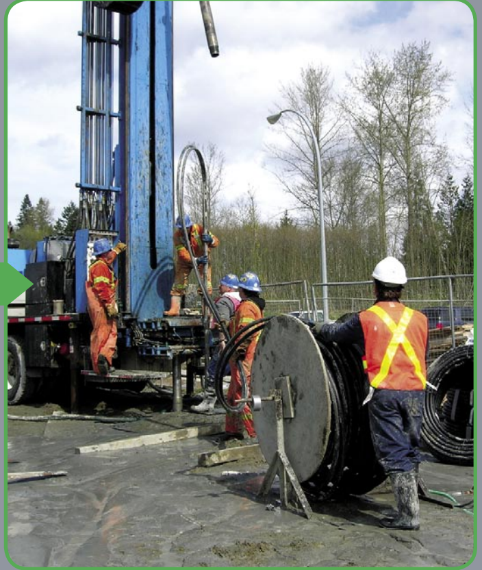
■ Lowering of geo loop.
