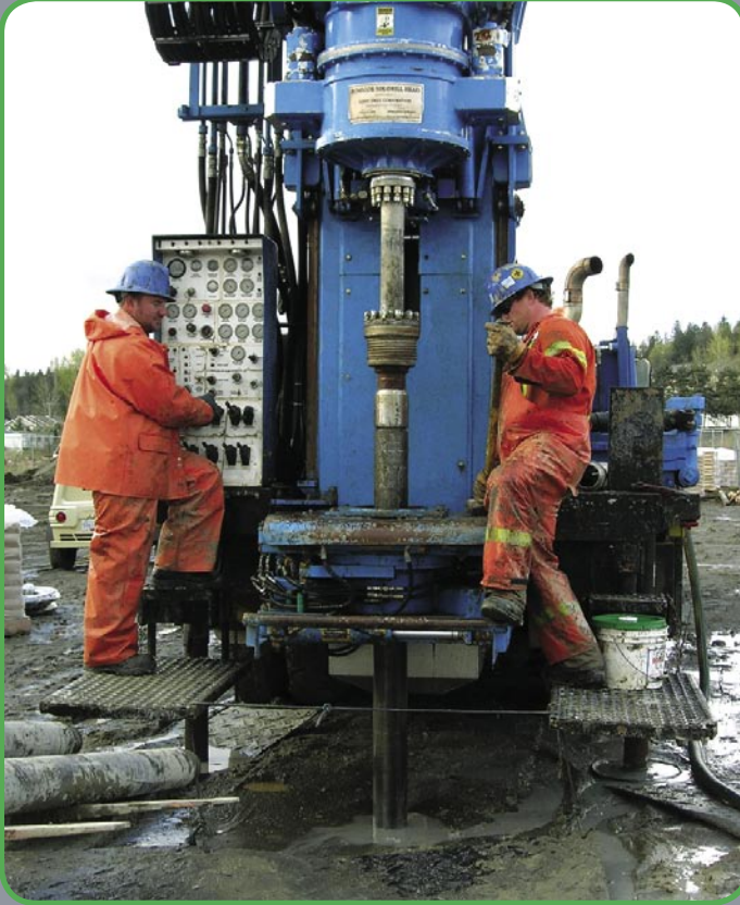
■ Drilling in progress.
