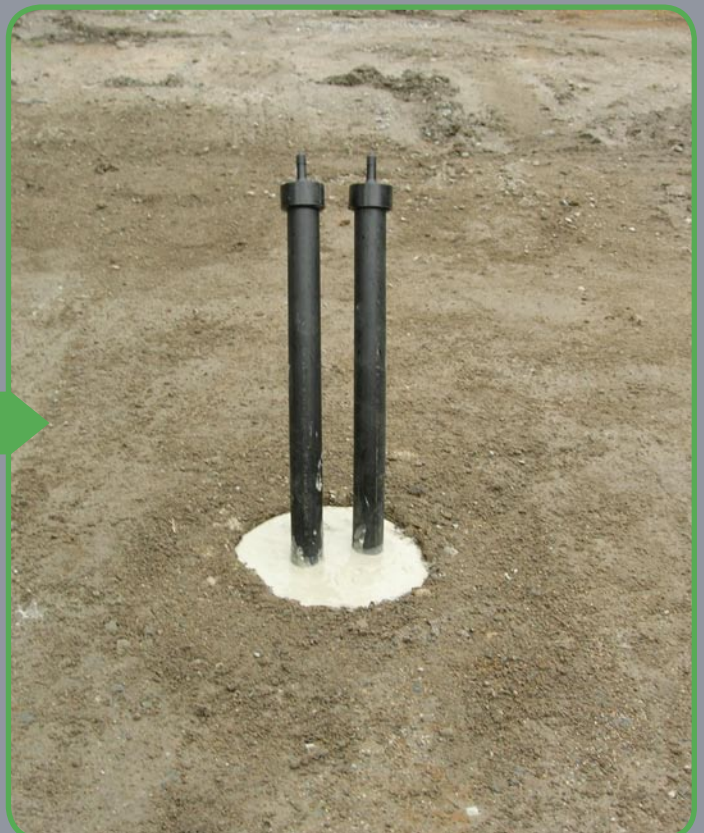
■ Completed geo loop installation.
