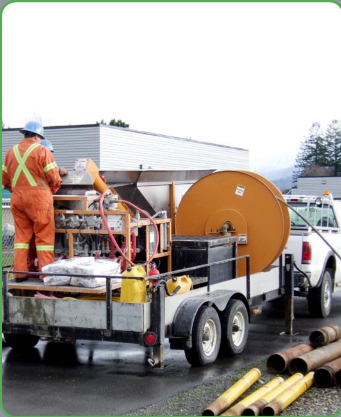
■ Grouting of geo loop.
